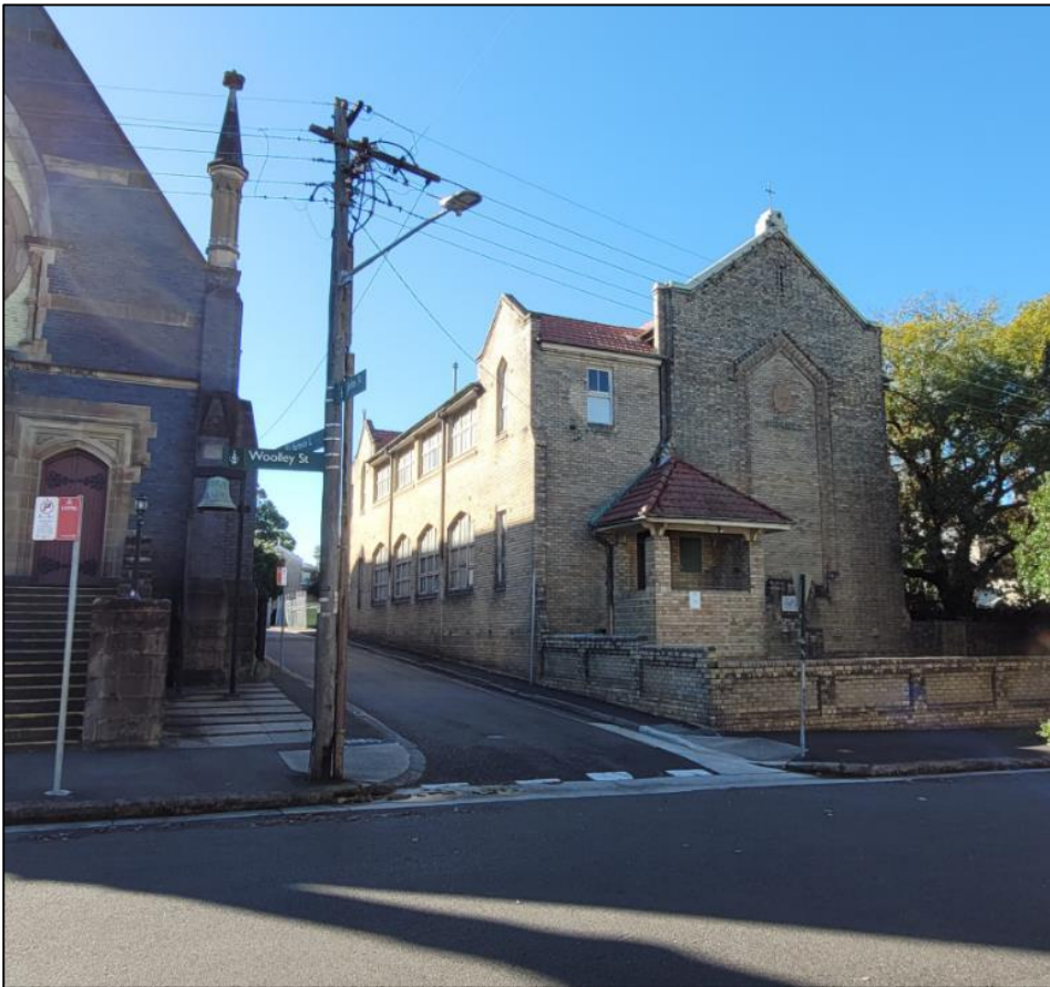
Figure 36: View from west side of Woolley Street
