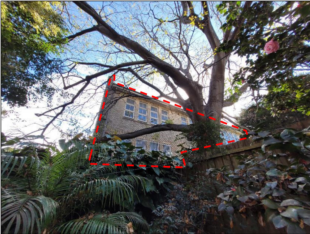
Figure 16: View from the rear yard of No.171 Bridge Road looking north towards the southern elevation of the parish building
