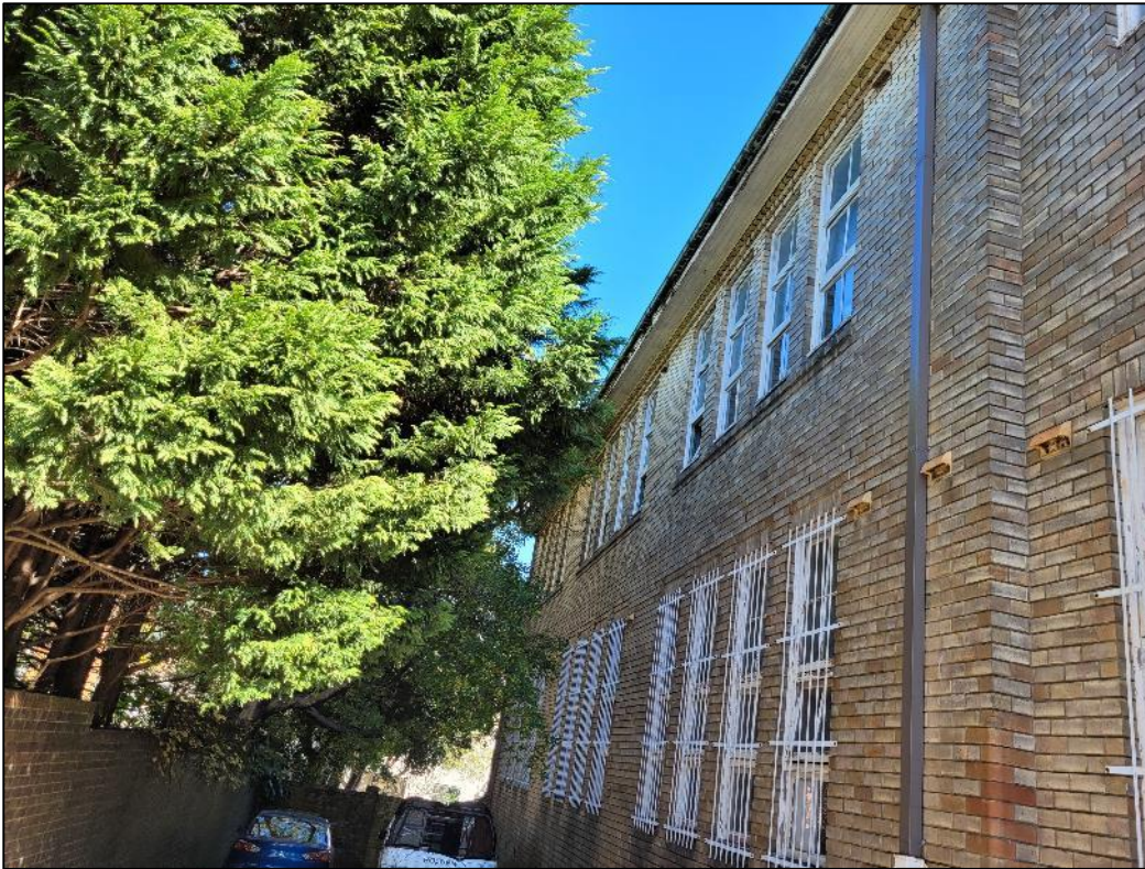
Figure 6: South-eastern elevation of the parish building
