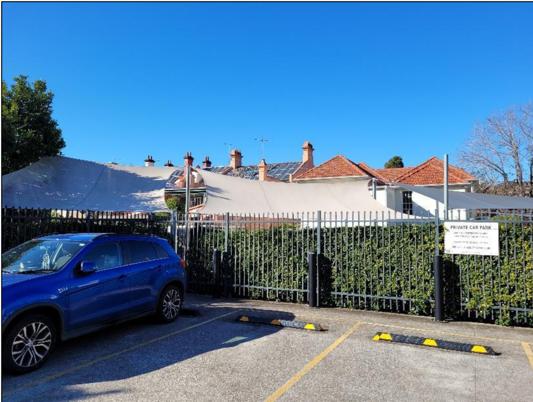
Figure 8: View from the car park looking south-east towards the child care centre
